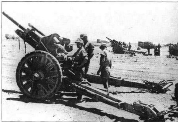
A leichte Batterie equipped with 105mm leichte Feldhaubitze 18 howitzers is ready to open fire (note the 3-ton Hanomag H kl 6 SdKfz 11 half-tracks in the background). This howitzer was inferior to its British equivalent, the 25-pdr. (Carlo Pecchi Collection)
